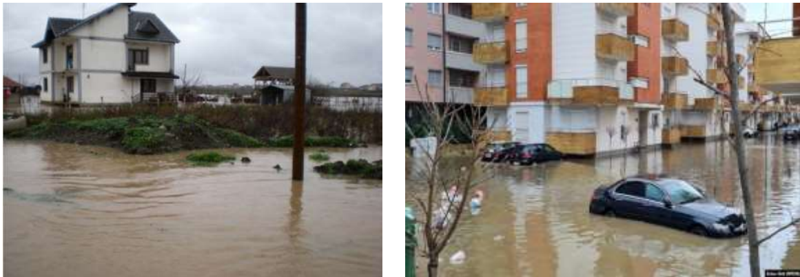
Figure 26: Road status after floods in 2010
